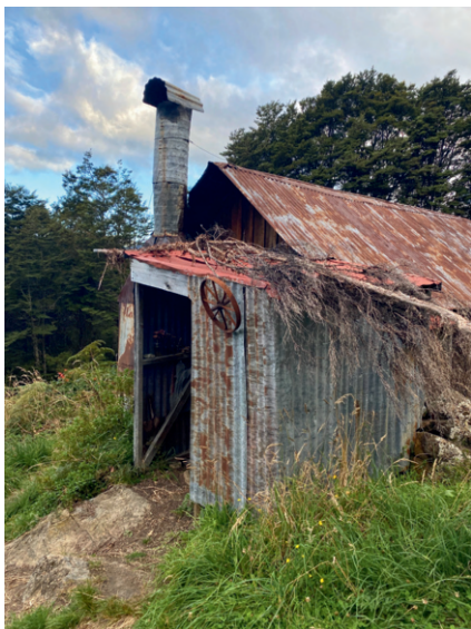
Asbestos Cottage in Kahurangi National Park. Slightly scary, full of character.
