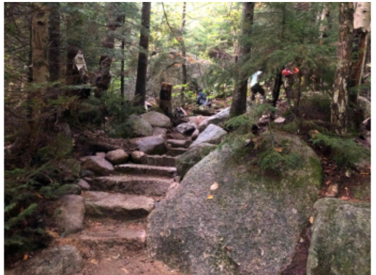
OBP in WHNF Fall 2022 - Trail condition before and after with new stone steps and edging, filling the eroded gully and making a wider footpath
