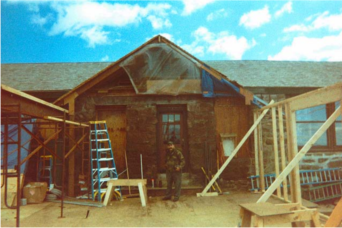
Madison Hut Renovation – 9/21/2010
